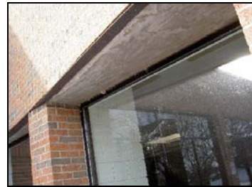
Structural Header
