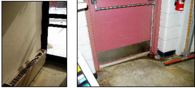
Figure 3.24 Engineering Tech – Air Infiltration Through Entryways
