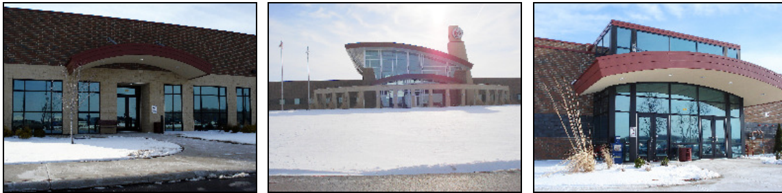
Figure 3.34 Findlay Campus – General Views of Buildings
