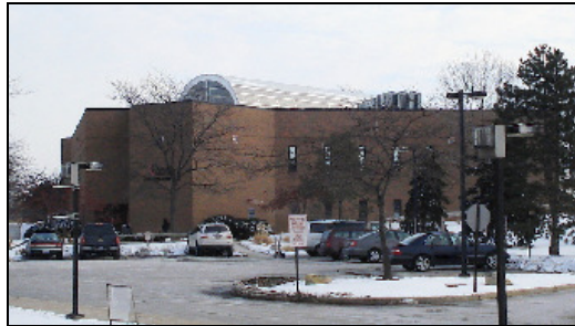
Figure 3.20 Administration – Limited Exterior Glazing
