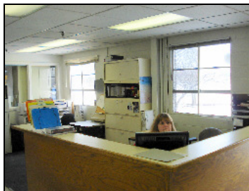
Figure 3.32 Facilities – Single Glazed Windows
